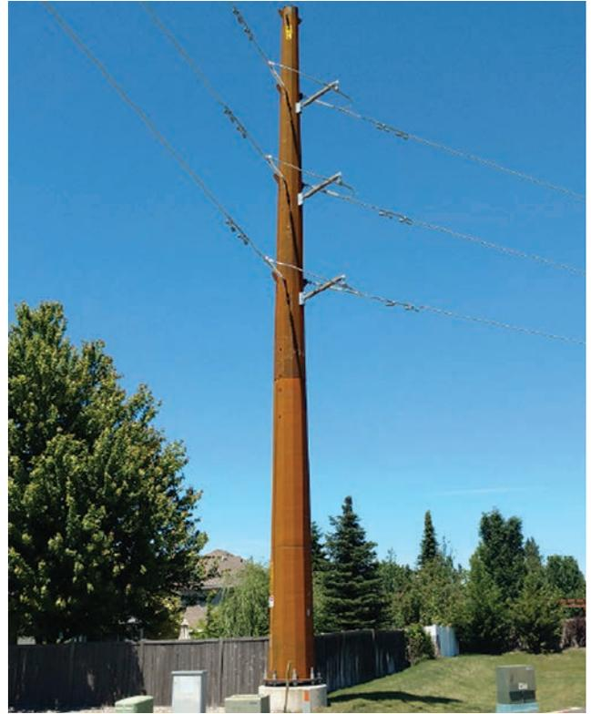
EX3 Technology enabled the replacement transmission line to have 15% higher line ratings. The new line uses fewer, but taller, self-weathering steel poles.
