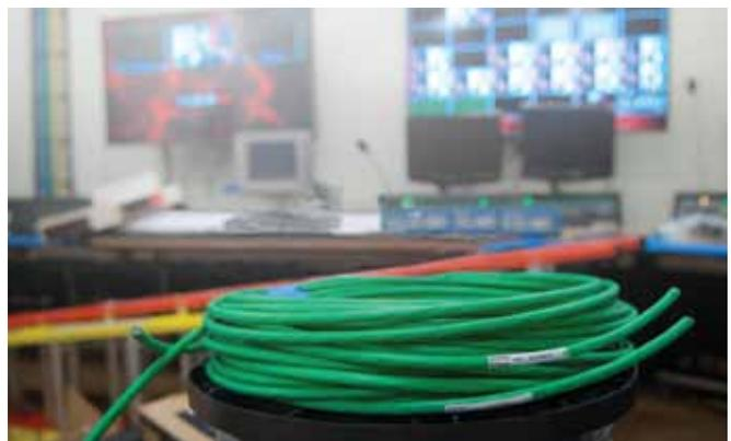
**The PanGen system installed in Griffin Hall comprises General Cable's GenSPEED 10 Mosaic Twisted Pair Category 6A cable, shown here, and connectivity from Panduit, for cabling channels certified to support 10-Gbit Ethernet.**
