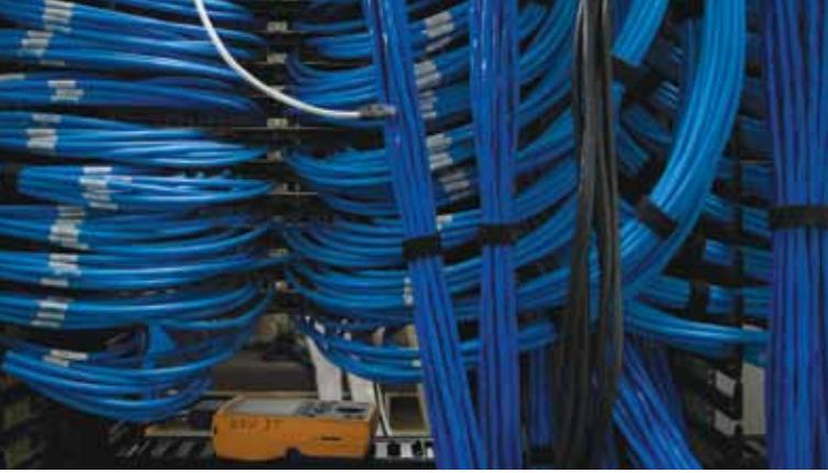
**Inside a rack within one of Griffin Hall's telecommunications rooms. In total, the building includes approximately 3,000 work area outlets. In high-tech classrooms, anywhere from 24 to 36 connections were installed in the floor and another 40 in the wall.**
