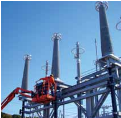
Commissioning Test Preparation
